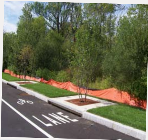
The use of native plants enhances pollutant removal and appearance along the street.
