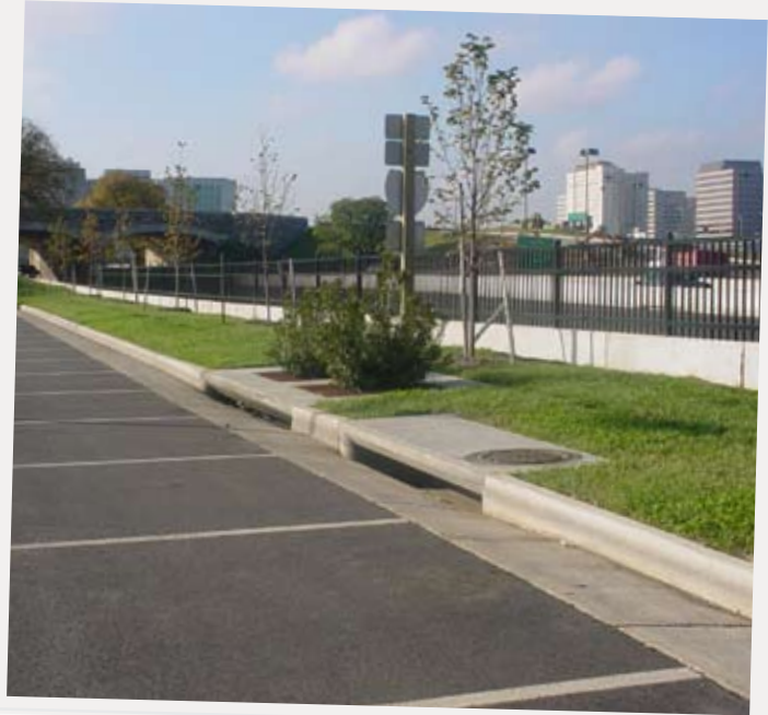
Filterra installations along the secure bypass at the U.S. Pentagon met local stormwater quality regulations, protecting the Potomac River and Chesapeake Bay watershed.
