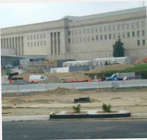
Filterra units placed within the roadways increased buildable space to maximize parking.
