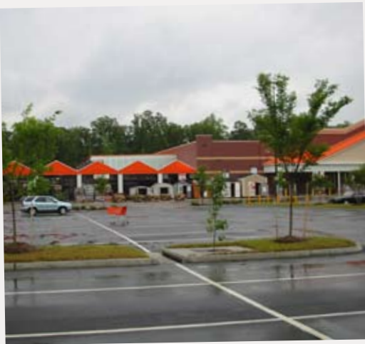
Placing Filterra within traffic islands maximized customer parking and enhanced the landscape.
