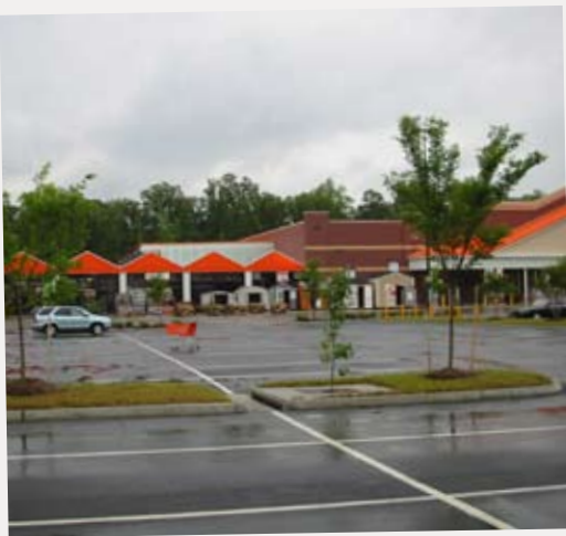
Placing Filterra within traffic islands maximized customer parking and enhanced the landscape.
