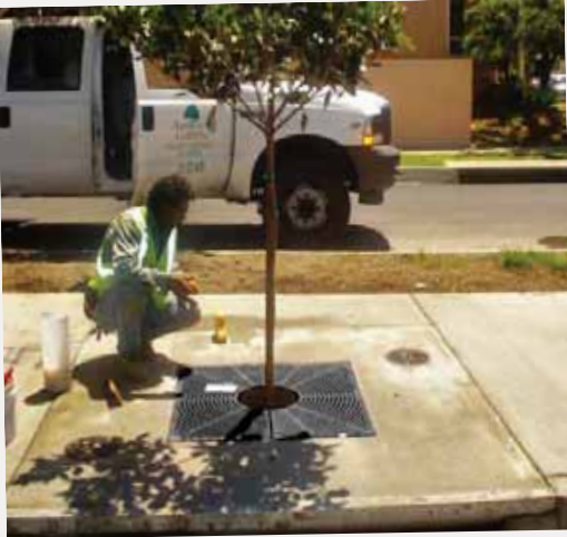
Filterra's small footprint made for simple installation along Paramount Boulevard.
