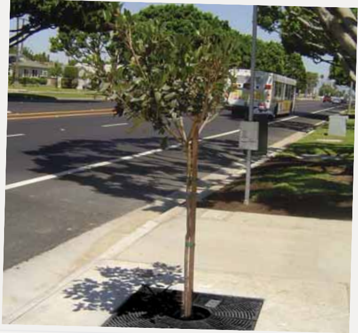
One of several Filterra Bioretention Systems installations along the Paramount Boulevard corridor.
