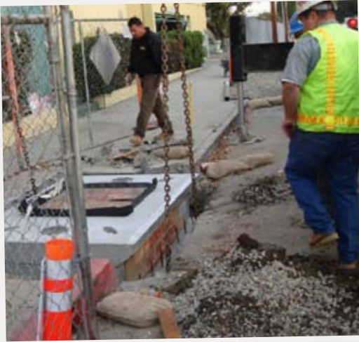
Filterra's small footprint made for simple installation on Marina Del Rey streets.
