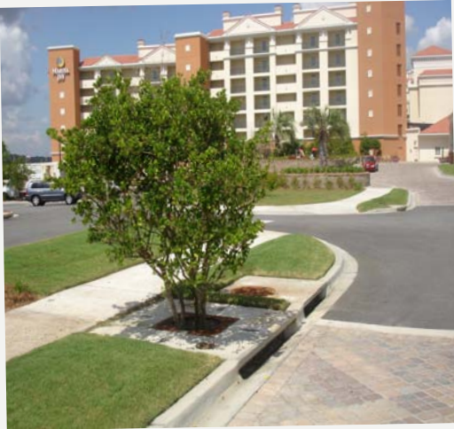
Filterra was installed to meet Federal, state and local stormwater requirements, as well as to enhance property value and increase buildable space.
