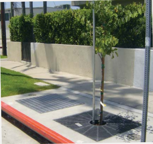
Filterra's small footprint made for simple installation along Grand Boulevard in Venice.
