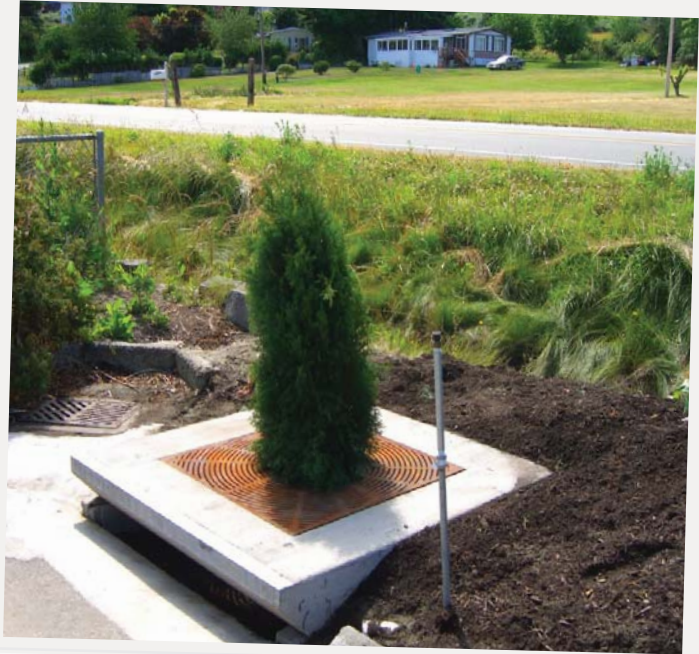
A Filterra Bioretention System was installed at Freeland Park to help treat urban runoff, reducing the amount of pollutants entering Holmes Harbor.
