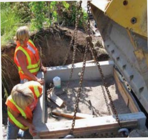
Filtrerra's small footprint made for simple installation in Freeland Park.
