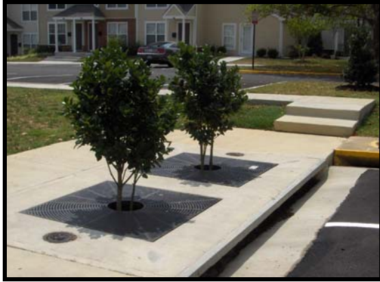
Figure 2 (left) – Hollies planted in Filterra ® units installed in a parking lot with replicate landscape holly in background. Figure 3 (right) – Collection of leaves from a holly for N and P analysis.
